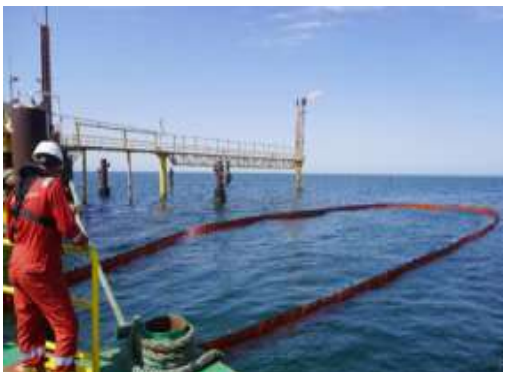
Containment of the oil spill - 21.09.2023
