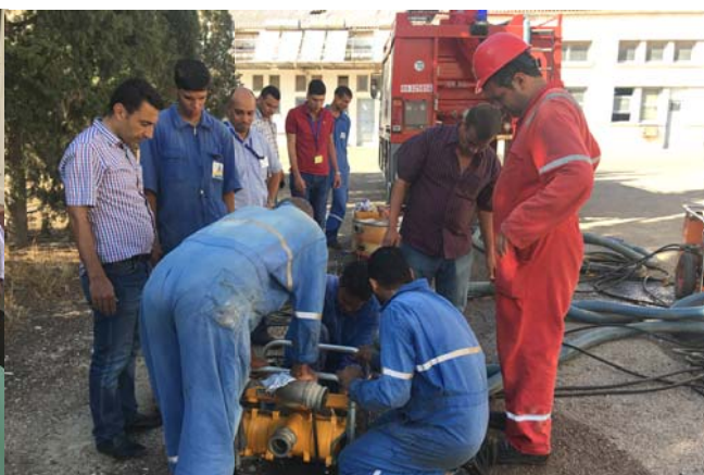
Maintenance of Pump
