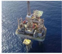
contiguous to a drilling and production jack-up "Jawhara 5", a loading vessel Floating Storage Offloading (FSO) "Thapsus", a 1400 meters underwater pipe (sealine) for the transfer of oil production from the platform to the loading vessel, and a mooring buoy (CALM Buoy).
